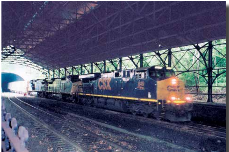
Single stack train emerging from the tunnel.
