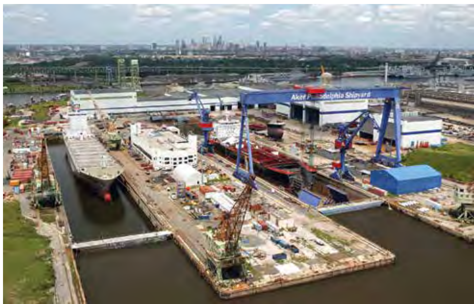
A ship under construction at Philly Shipyard (formerly Aker Philadelphia Shipyard). According to the Wall Street Journal, the yard has delivered more than half of all Jones Act oceangoing vessels since 2003. It has recently obtained orders from MARAD for repairs to Ready Reserve ships, but it needs new ship orders to keep its workforce employed. PHOTO COURTESY OF PHILLY SHIPYARD
