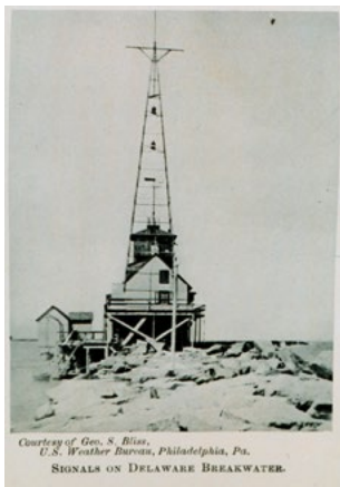
Courtesy of Gen. S. Biles, U.S. Weather Bureau, Philadelphia, Pa. SIGNALS ON DELAWARE BREAKWATER. Picture 1 - Signal Tower for Storm Warning Flags used by day, lanterns by night. Used to warn mariners in: "The Boy and the U.S. Weather Men", 1917, p.236. Photo Courtesy of U.S. Weather Bureau circa 1910.
