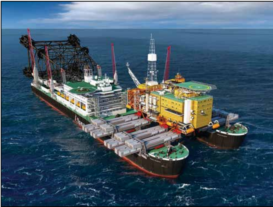
Launched in 2013, the MV Pioneering Spirit is the worlds largest construction ship, designed for the single-lift installation and removal of large oil and gas platforms. 1565' LOA, 407' Beam, 403,342 GT
