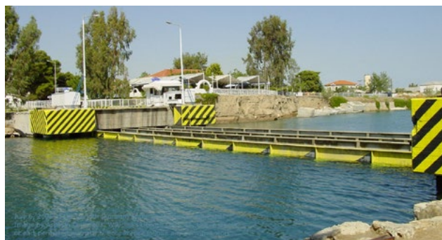
Submersible bridge at the Corinth entrance to the Corinth Canal.
