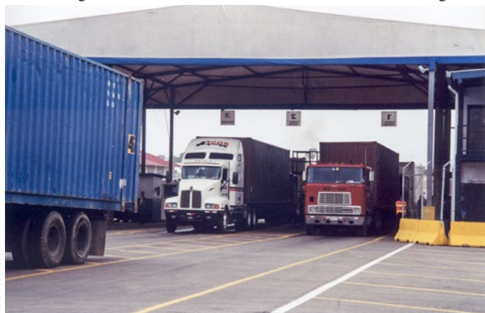
Truck security gate at the Manzanillo International Terminal (MIT) facility in Panama.
