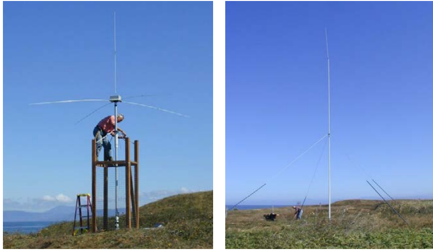
Figure 2: The antennas for (a) receiving and (b) transmitting radio waves at each site.
