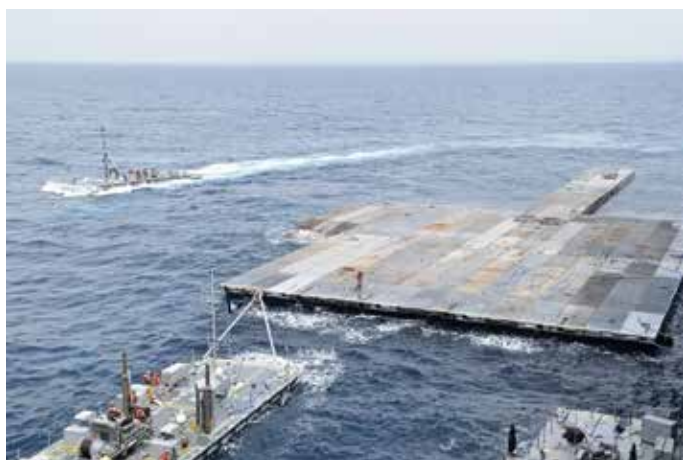
The Trident Pier under construction. The US military said the floating pier would be able to handle 150 lorry loads of aid per day once fully operational. The pier is part of the US's Joint Logistics Over the Shore capability
